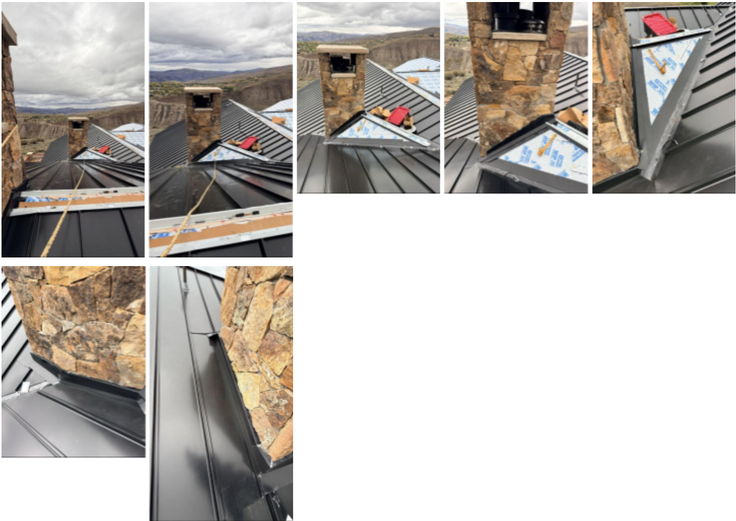
Description/Notes: Flashing is being completed now
