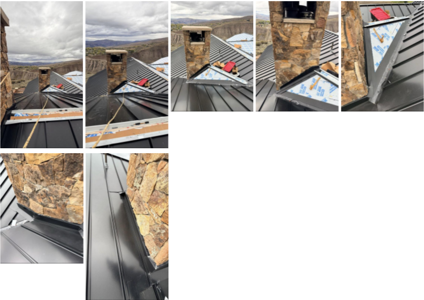
Description/Notes: Flashing being completed.
